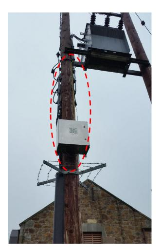
Figure 6 Receiving station 1 mounted on OHL pole
