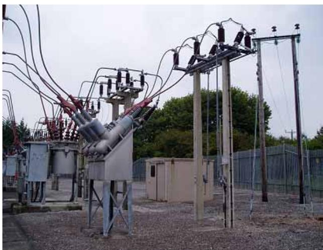
Figure 9. Side photograph of the ABI, VCB and substation building
